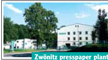
Zwönitz presspaper plant
